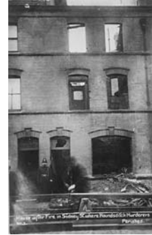
47 The House after fire in Sidney st.
